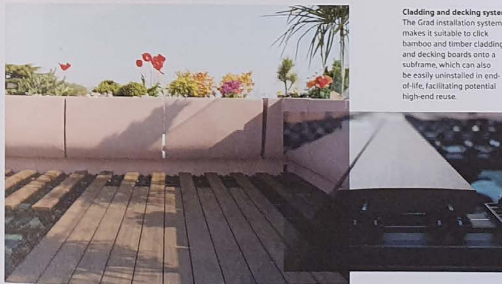
CLT and bamboo house The family home of architect Bart Spee (designed by Spee Architecten) is made of a CLT shell and finished with thermally modified bamboo (Bamboo X-treme) for the façade and roof cladding, installed on a demountable rail system to facilitate reuse in end-of-life.
