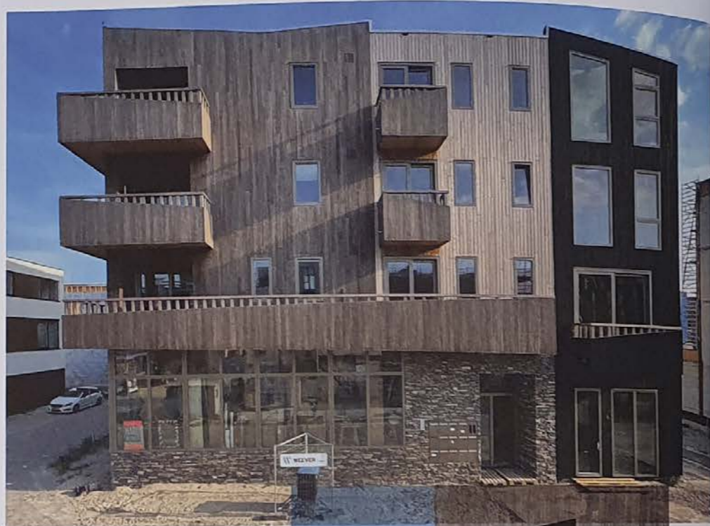
Multi-story CLT building The apartment building Mooliburg in Amsterdam (designed by Natruflief Architecture) features a CLT bearing structure and is finished with thermally modified softwood and thermally modified bamboo both in regular form (Bamboo X-treme) and partly with a charred surface (yakisugi finishing). Due to the compression, the bamboo reaches Euro-class B regarding fire safety and does not need additional impregnation with fire retardants.
